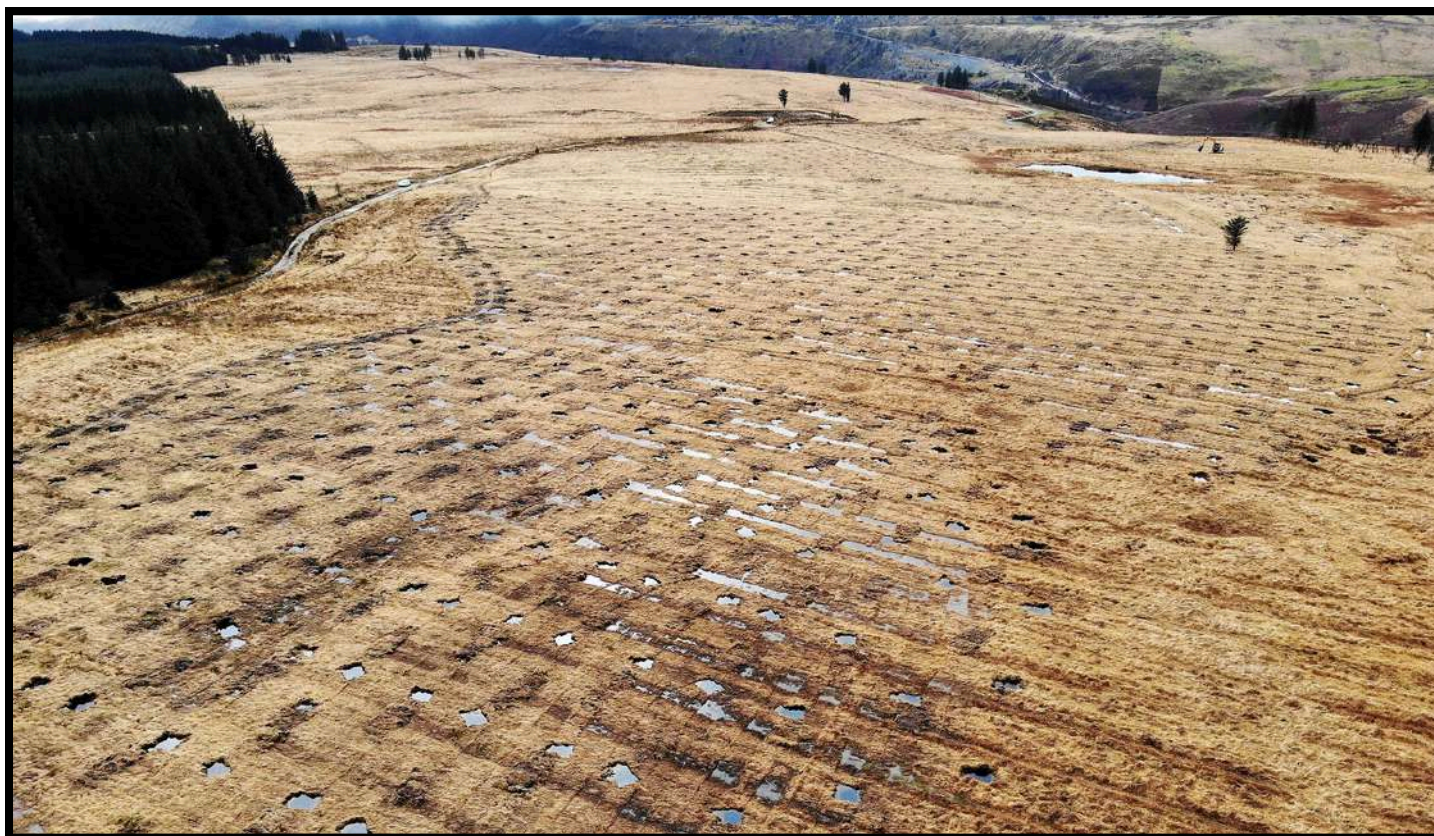
Castell Nos RCT: After restoration - peat dams blocking drainage channels
